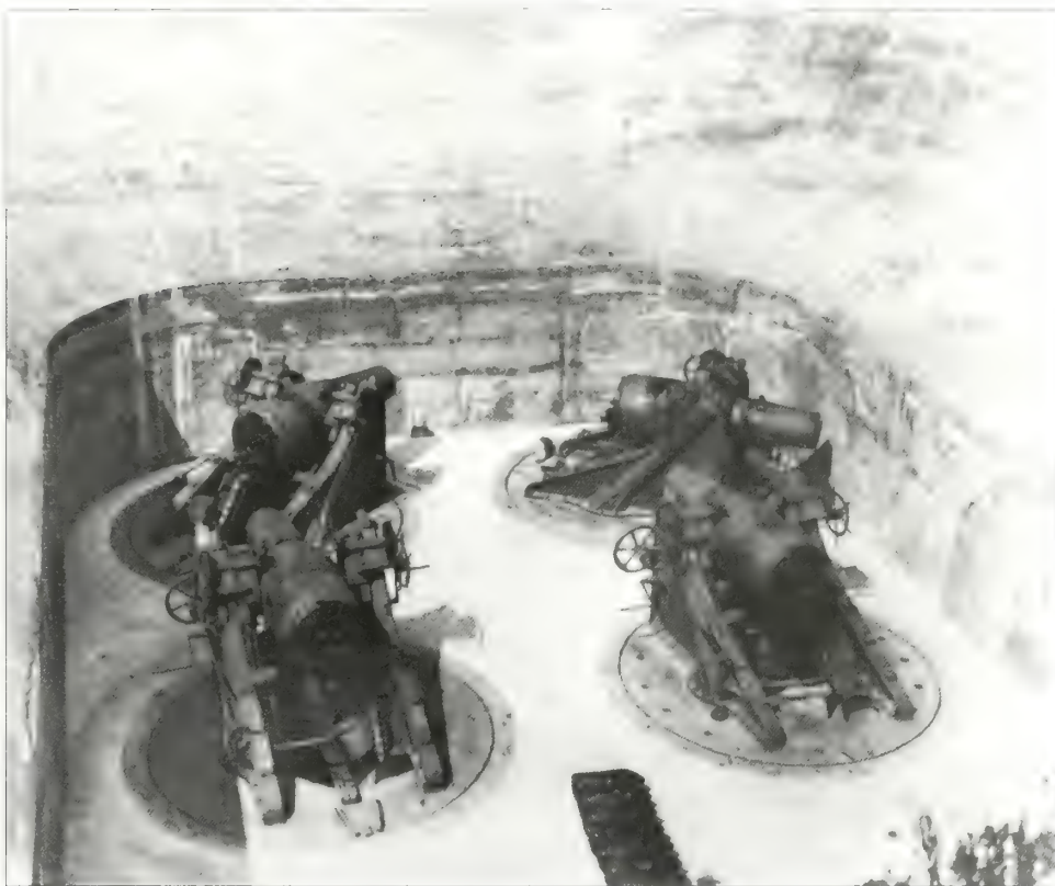
Figure 2.18. Four mortars mounted in a mortar pit, the Mortar Battery, June 30, 1894. Compared to the long-barreled guns at Battery Potter, mortars were stubby and set at steep angles to fire their projectiles in a high, arcing trajectory (GATE 7864).
